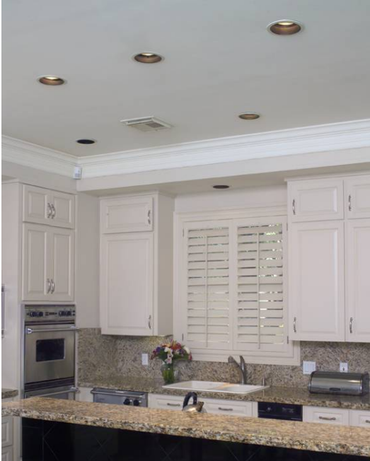
Existing recessed lighting.
