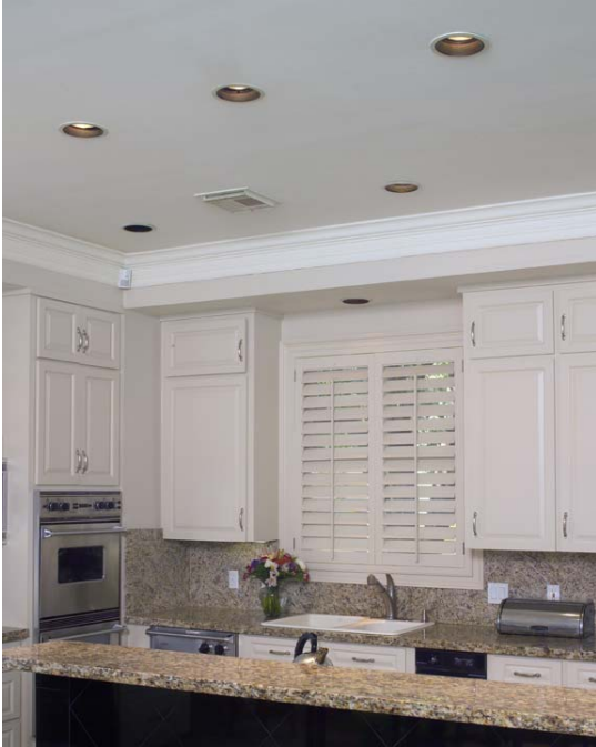
Existing recessed lighting.
